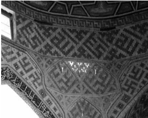
Figure 15: The broken lines at the edge connected to the interior of the dome, Great Mosque
