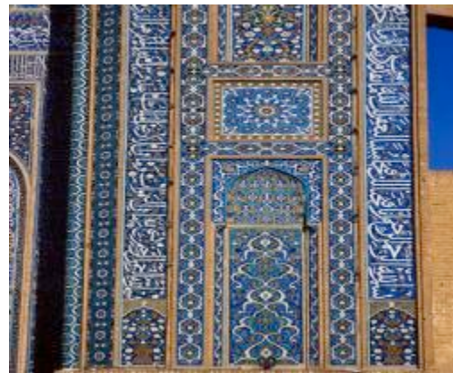
Figure 10. The motif of the triangle, the south porch tiles, Great mosque
