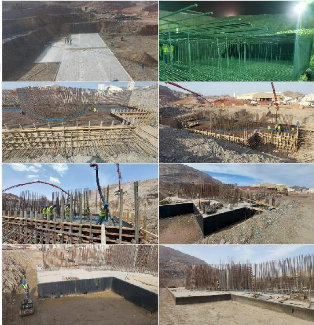
Figure 4-2 On-Site Observations for Plain Concrete, Foundation, & Backfilling.
