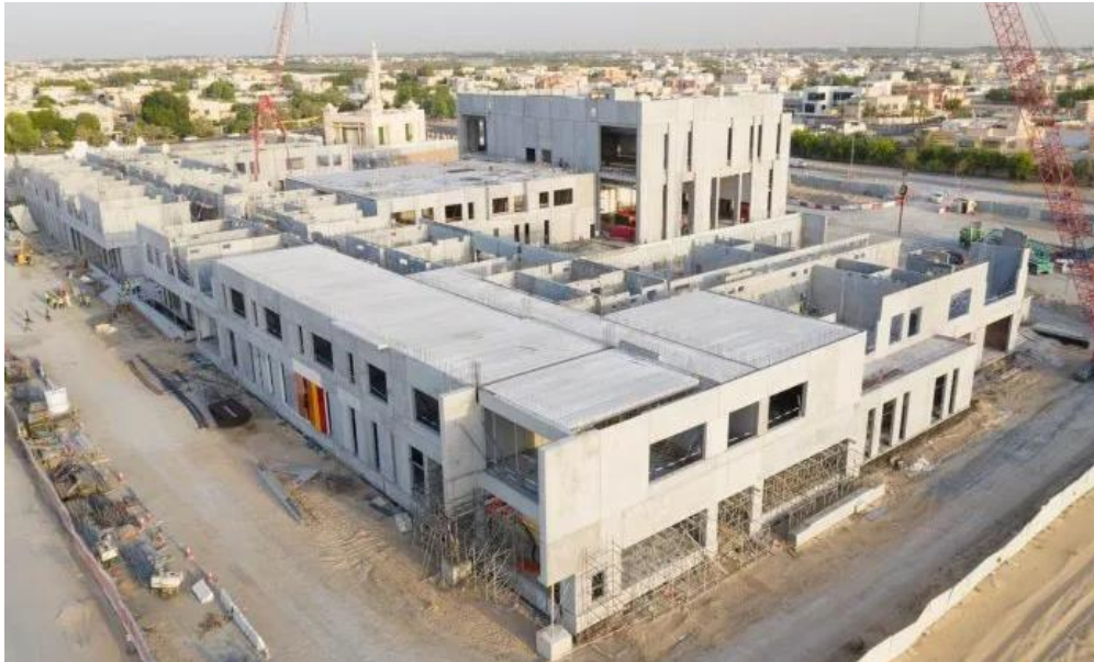
Figure 2.4: Prefabricate concrete project
