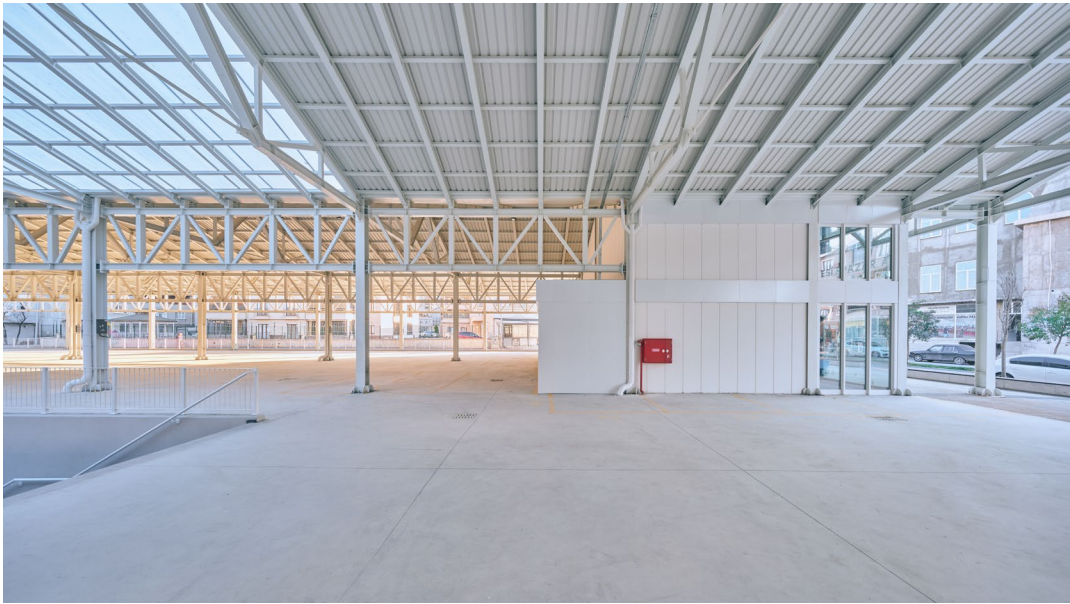
Figure 9: Millet Covered Bazaar, cellular concrete wall panels between the steel structure (Per Se Architecture, 2022).
