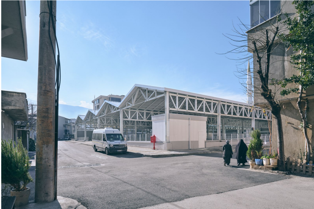
Figure 8: Millet Covered Bazaar, cellular concrete wall panels forming load-bearing walls (Per Se Architecture, 2022).
