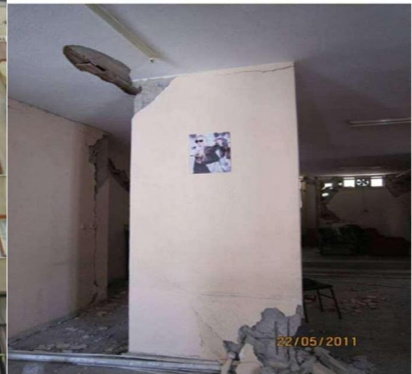
(b) Interior damage on the column during pounding
