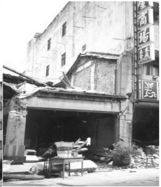
(b) Collapse building due to pounding
