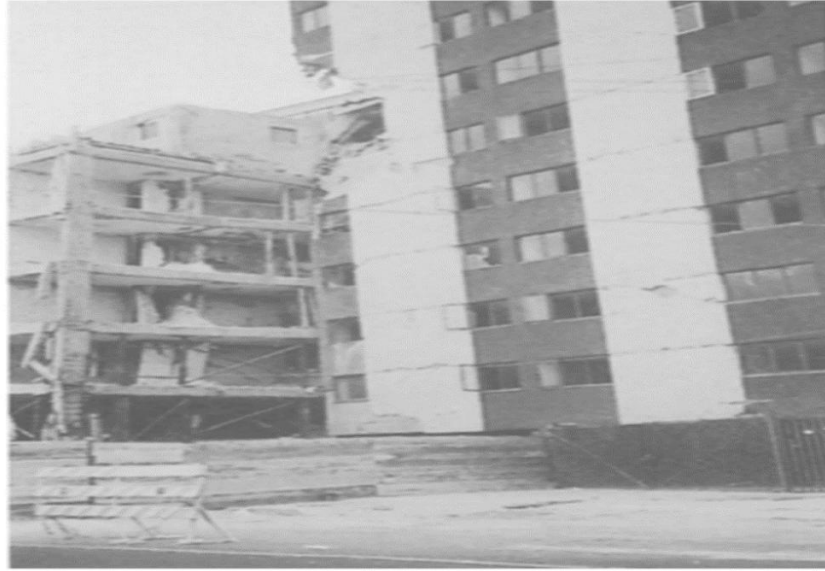
Figure 1.2: Pounding damages of adjacent buildings during the Mexico earthquake (1985) [4].
