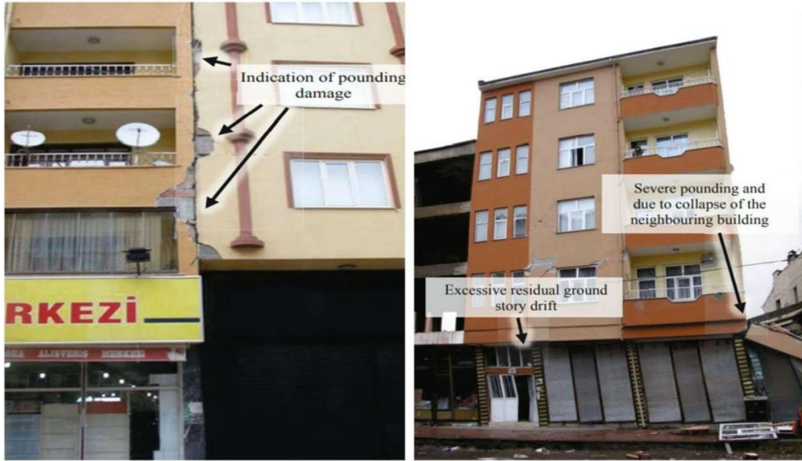
(a) Van buildings affected by pounding
