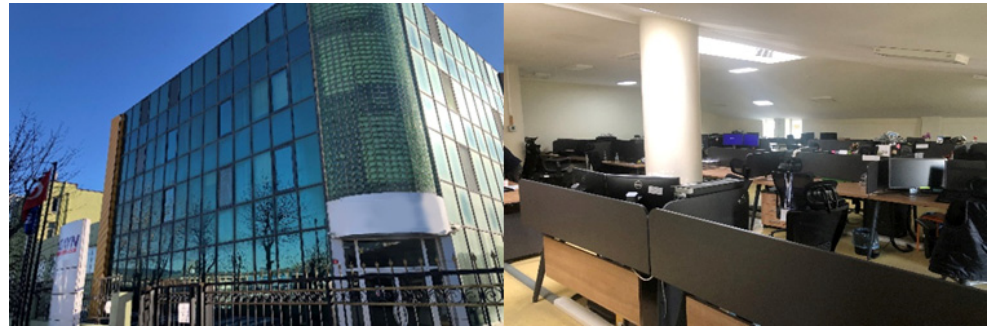
Figure 1. Exterior and interior views of the building.
