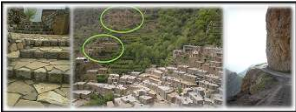
Picture 18 (left): beginning the pavement of pathways, picture 19 (middle): constructing new houses at the top of the village. Picture 19 (right): improper link road of the village to the cities (Source: authors).
