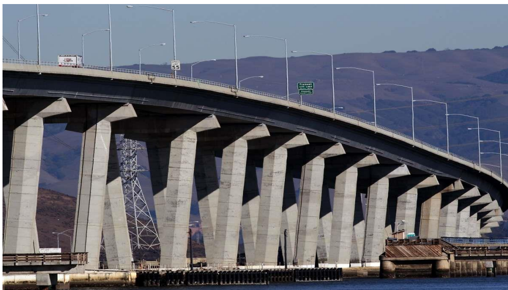
Figure 2.23: Dumbarton Bridge (Buffalo bridge) [31]
