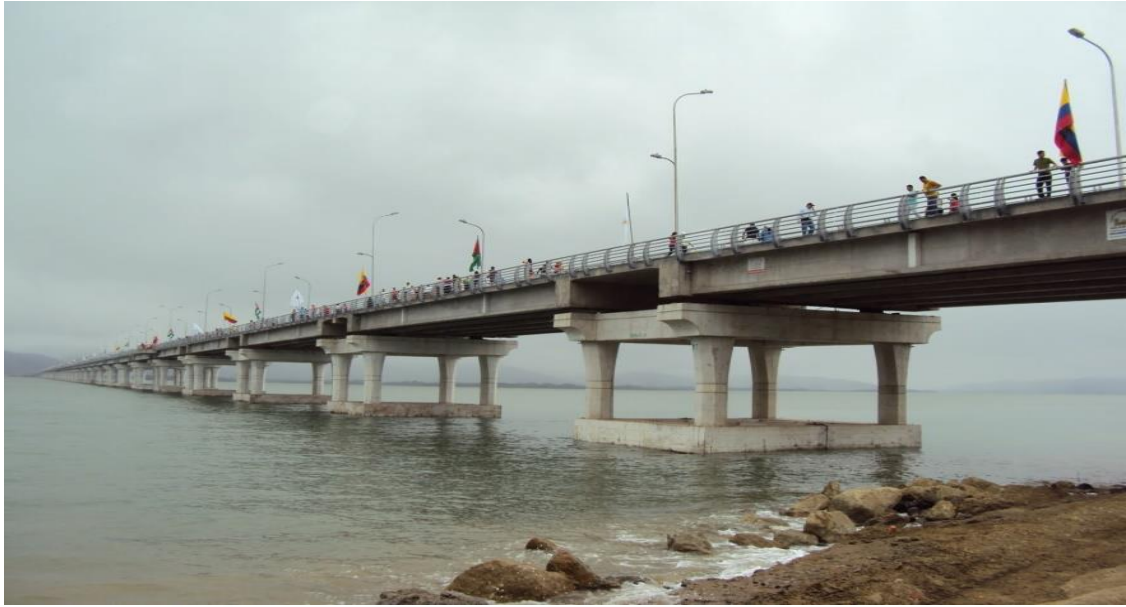
Figure 2.20: Los Caras Bridge [26]
