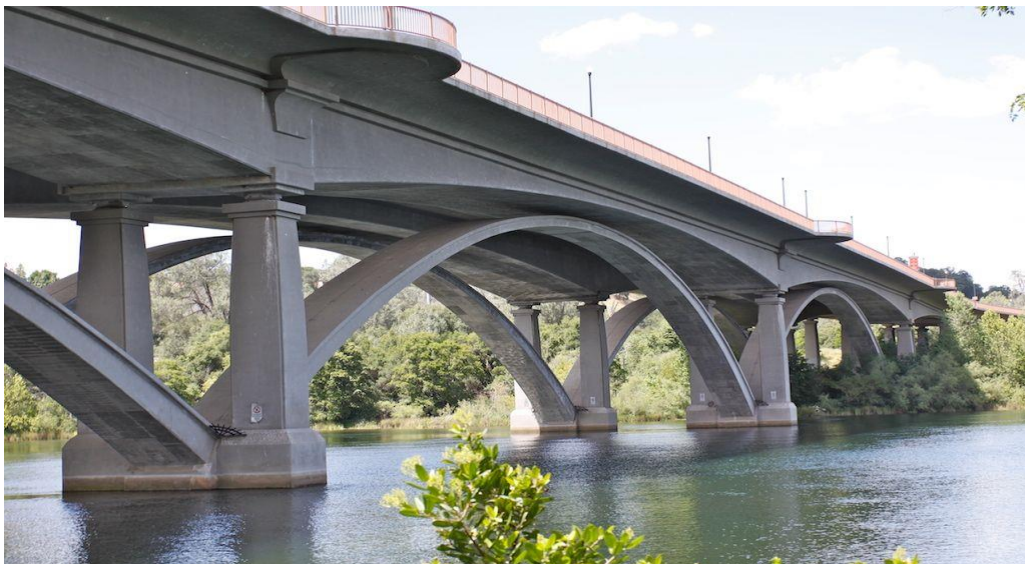
Figure 2.21: Lake Natoma Crossing Bridge (American River) [28]
