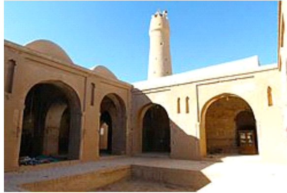
Figure 2. Fahraj mosque and simplicity in its architecture
