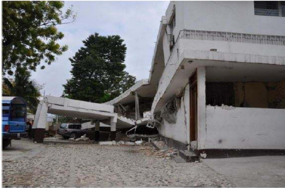
Figure 1.9: Building Damage during 2010 Haiti Earthquake
