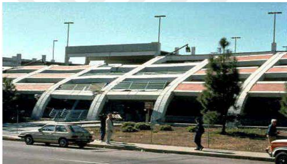
Figure 1.7: Failure of Parking Structure during Northridge Earthquake [4]
