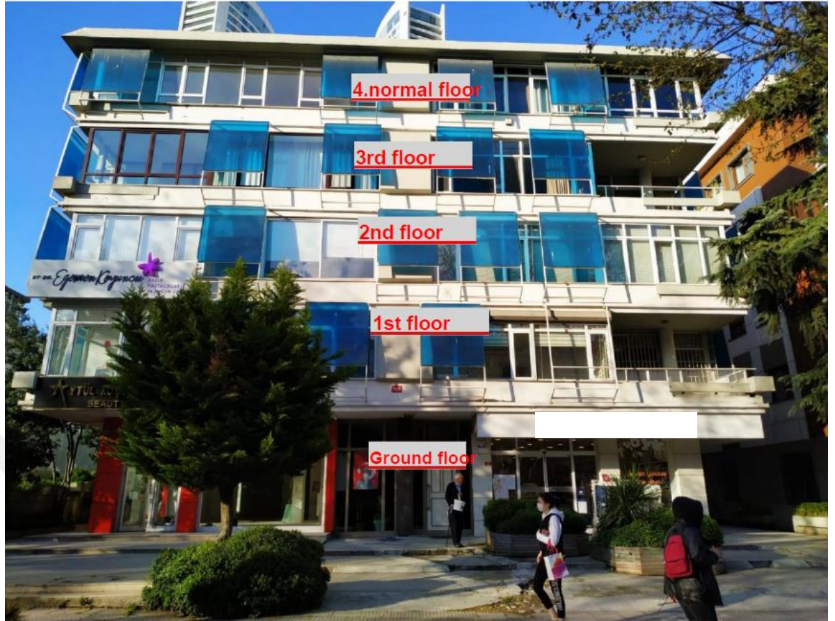
Figure 3.4 Building General view
