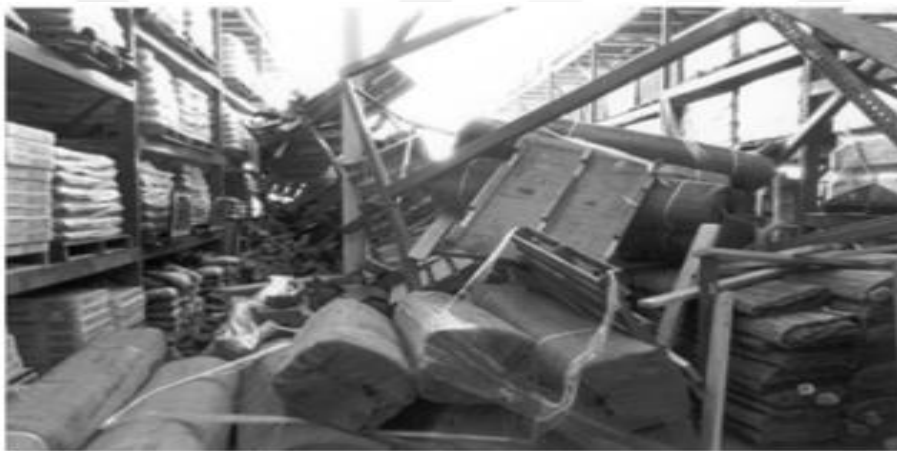
Figure 6: Collapse of a rack structure during earthquake at the Santa Clarita Store [2]
