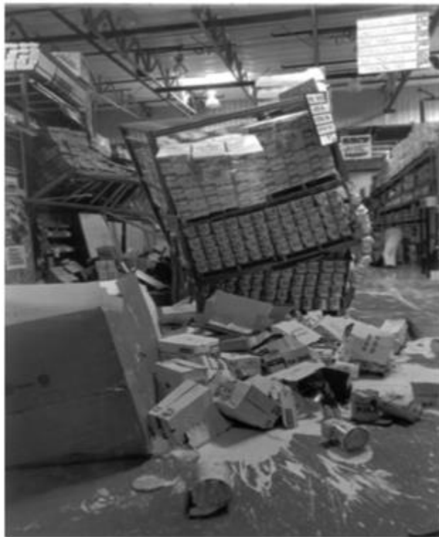
Figure 8: Collapse of a rack structure at the Santa Clarita Store [2]
