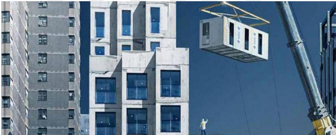
Figure 1 Residential units consisting of several modular boxes
