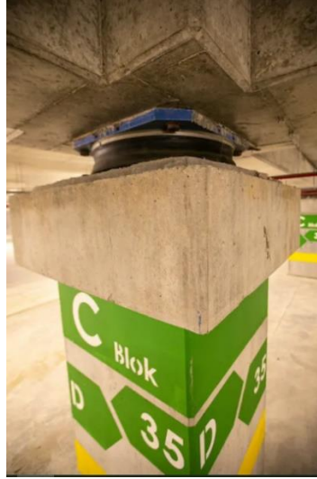
Figure 1.5: TFP installed in base floor (Reference)
