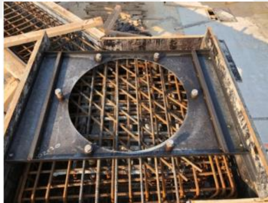
Figure 1.6: Foundation work for isolator installion (Yamanturk, Dogruoz, 2019)
