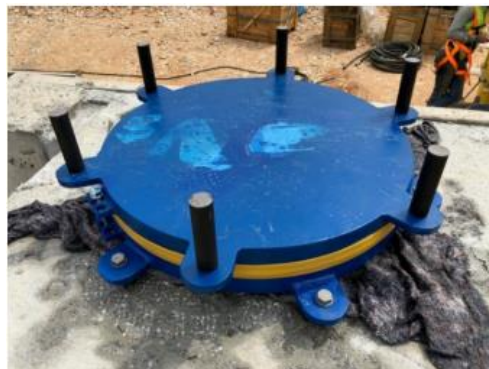
Figure 1.7: Installed double friction pendulum isolator view (Yamanturk, Dogruoz, 2019)
