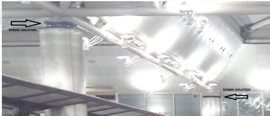
Figure 1.2: Seismic Isolation of terminal building
